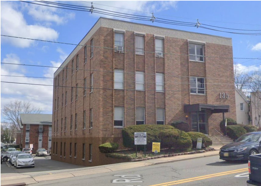
Photos of the site (Courtesy of Google, April and July 2022)
