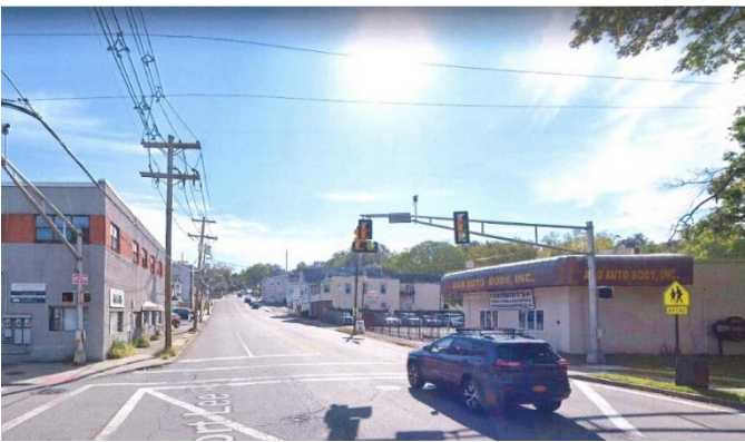
View of the existing conditions at the corner of Fort Lee Road and Willow Tree Road
