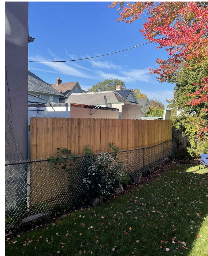
6 NEW SCREEN FENCE @ NORTH SIDE YARD (SOUTHWEST VIEW)
