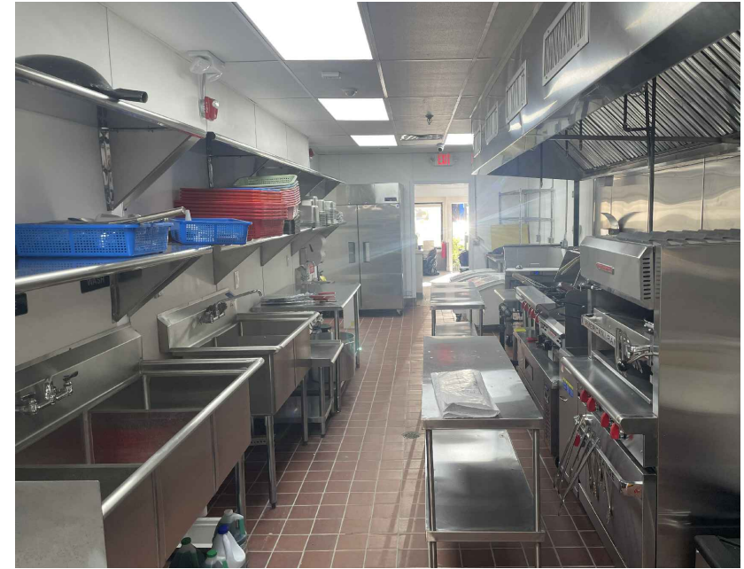
3 NEW KITCHEN FOOD PREP AREA
